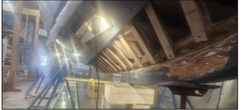
Repairing frames on LADY CLARE at Brooklin Boat Yard in Brooklin.
