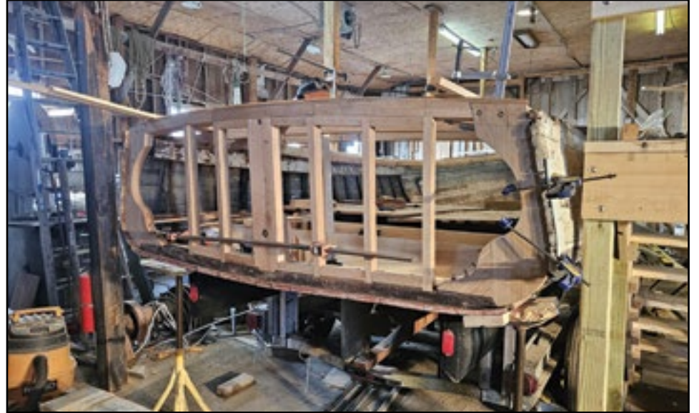
This is a stern view of the transom of the lobster boat CHRISTOPHER, which was built by Mariner and Isaac Beal in 1976. She is being rebuilt at Jonesport Shipyard under the guidance of Isaac Beal.
