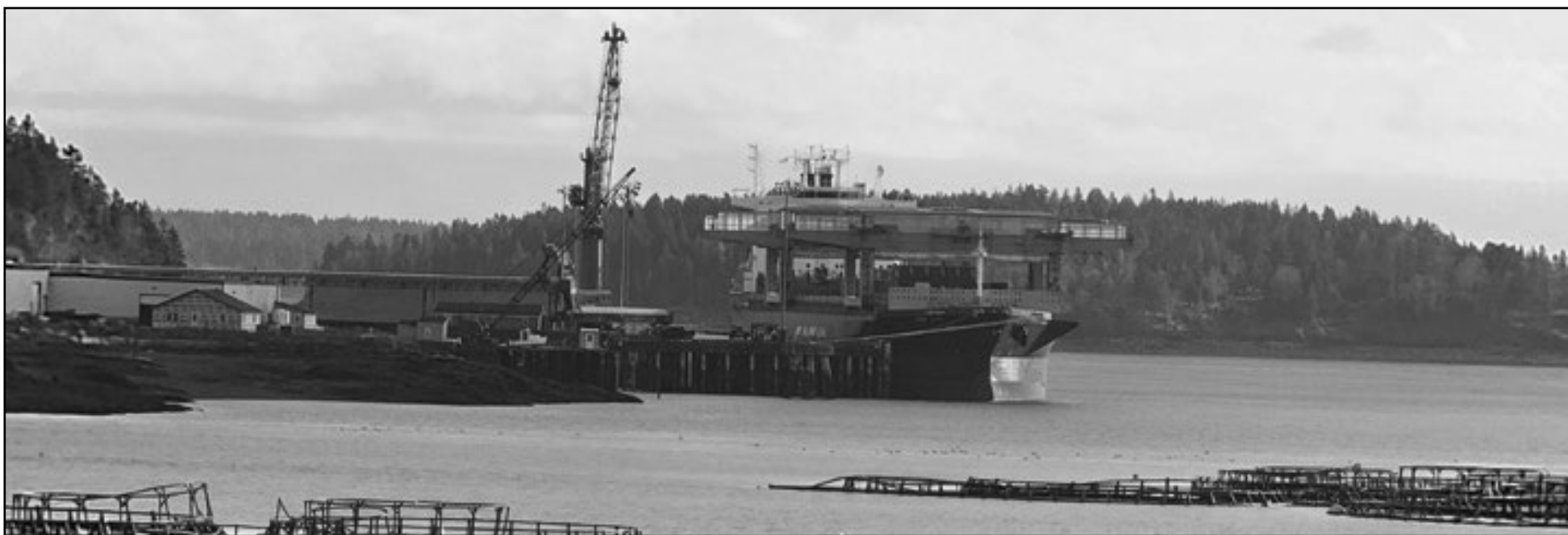
This is a cargo ship in at Estes Head in Eastport. This is the best port on the East Coast. It is the port closest to Europe, has a depth of 64 feet at the dock and never needs to be dredged.
