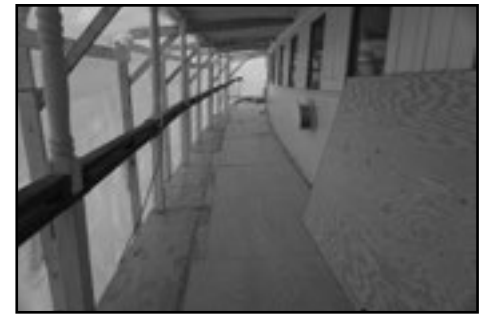
Port second level deck replacement.
