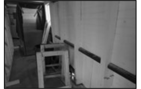
Pine bulwark planking above and below cap-rail. Framing also visible.
