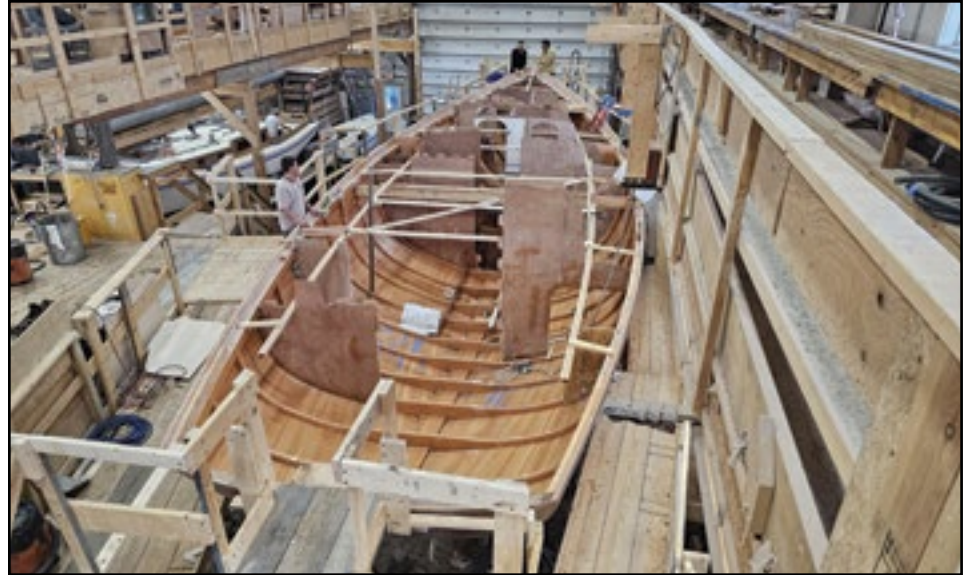
This is a 56-foot sailboat under construction at Brooklin Boat Yard in Brooklin. She has a cold-moulded hull, which was built upside down. Now that she is upright, they are now working on her interior.
