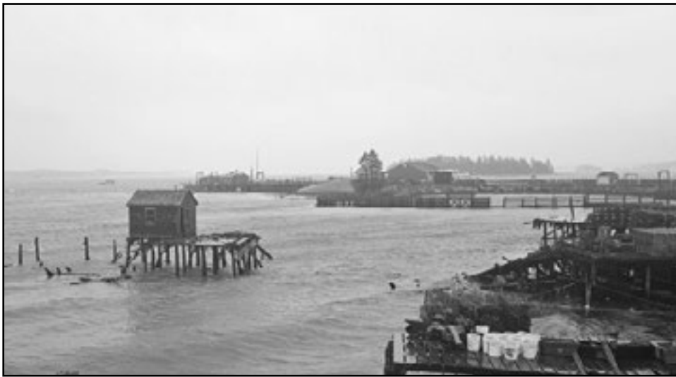
One of the fish piers on Beals Island suffers severe damage during the last big storm surge in January.
