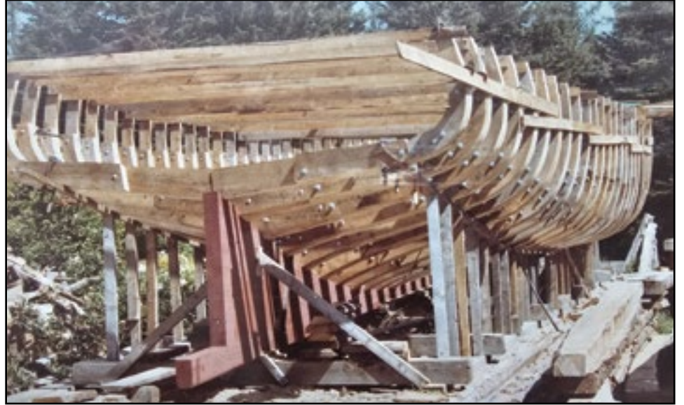
The hackmatack frames set up on the backbone set on her launching cradle.
