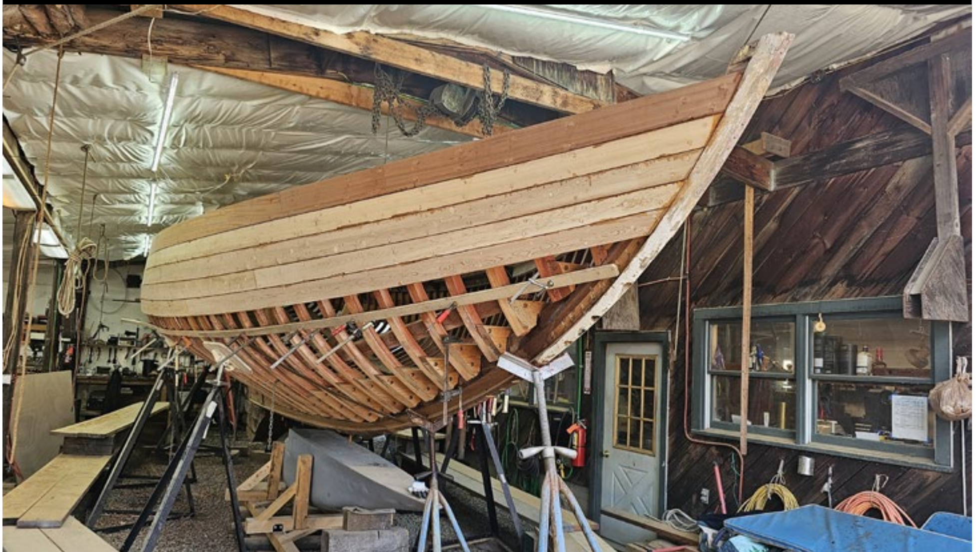
A 29-foot Concordia being totally rebuilt at Newcastle Marine in Newcastle.
