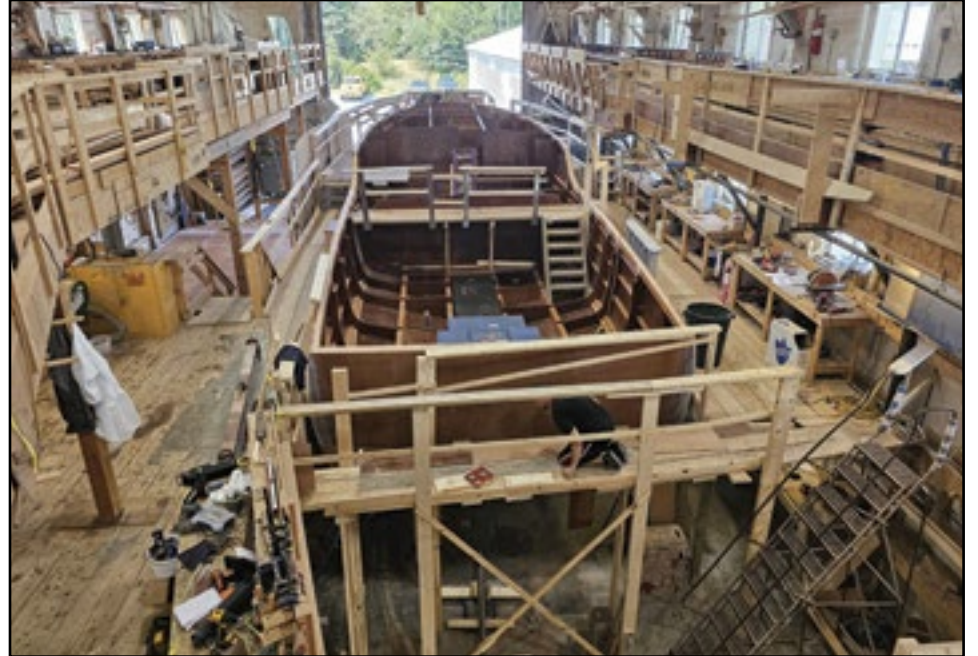
The 55-foot Wheeler hull has been rolled over and they are now putting in her interior structure at Brooklin Boat Yard in Brooklin.
