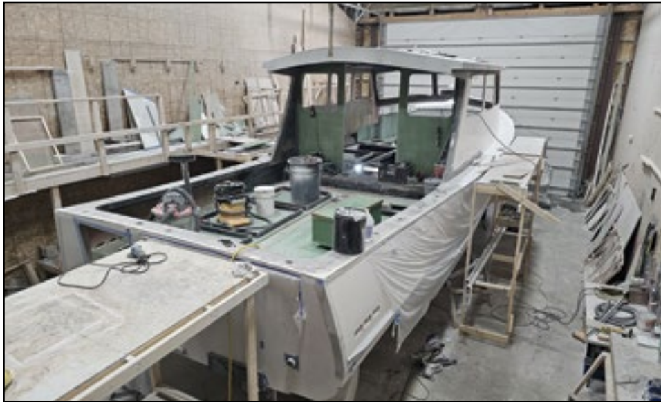
This is a Northern Bay 41 being finished out at Boricua Custom Boats in Steuben as a sport cruiser with a full interior. The engine is in and the interior has been roughed in.
